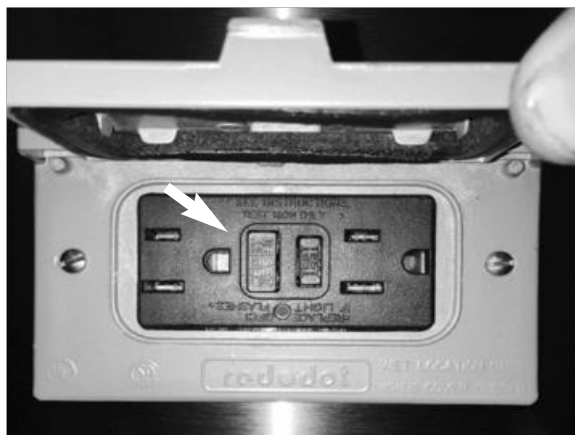
Figure 4-2. Reset Button on GFCI Outlet
