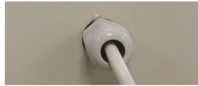
Figure 13. Schematic Diagram of Power Cord Access Port
