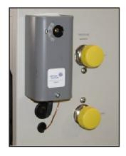
The monitor is not pre-set and must be adjusted during initial installation. The monitor is located on the rear of the exchanger.
